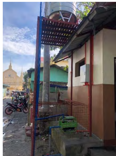
Figures 23 and 24: Solar-powered Water Pump at Public Market
